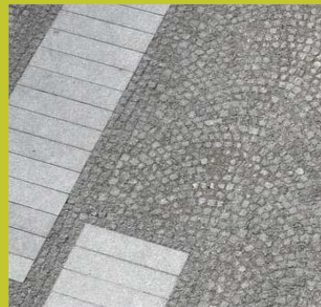
Paving cubes laid in 'Venetian Fan' pattern
