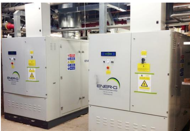
Figure 10: Example of CHP units
