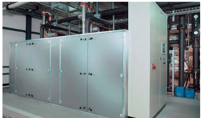
Figure 15: Typical water to water heat pump for GSHP
