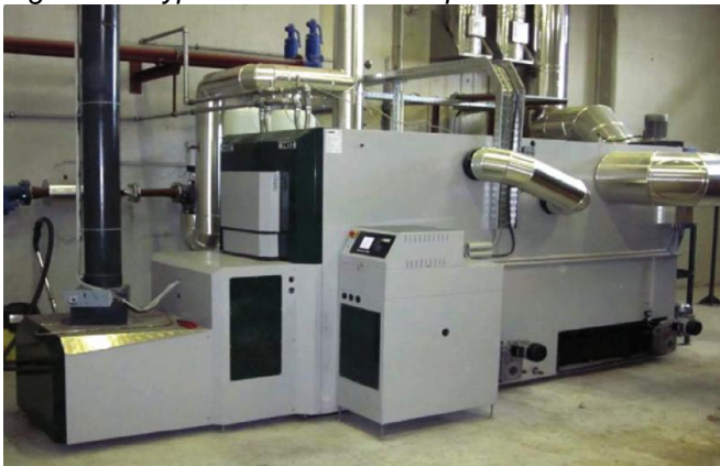
Figure 13: Typical Biomass boiler plant
