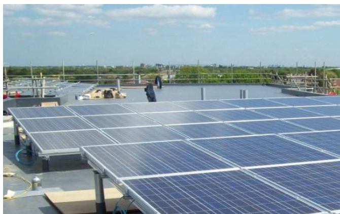
Figure 18: Typical PV installation
