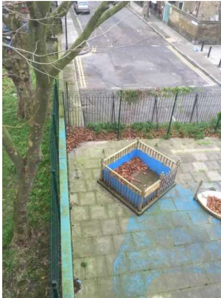
Image 4 – More roots were evident under the playground surface than public highway
