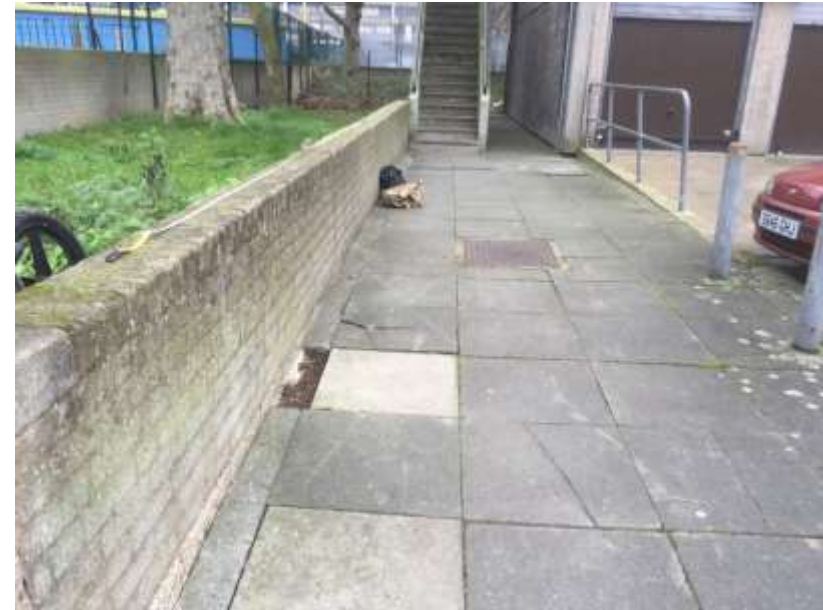
Image 3 – Roots were present in high numbers below hard standing but not below stairwell footing.
