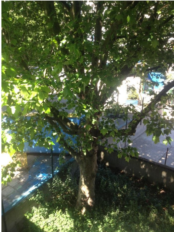
Image 2 – Shuttering and fencing to secure existing ‘soft’ ground areas where tree root radar work shows significant rooting
