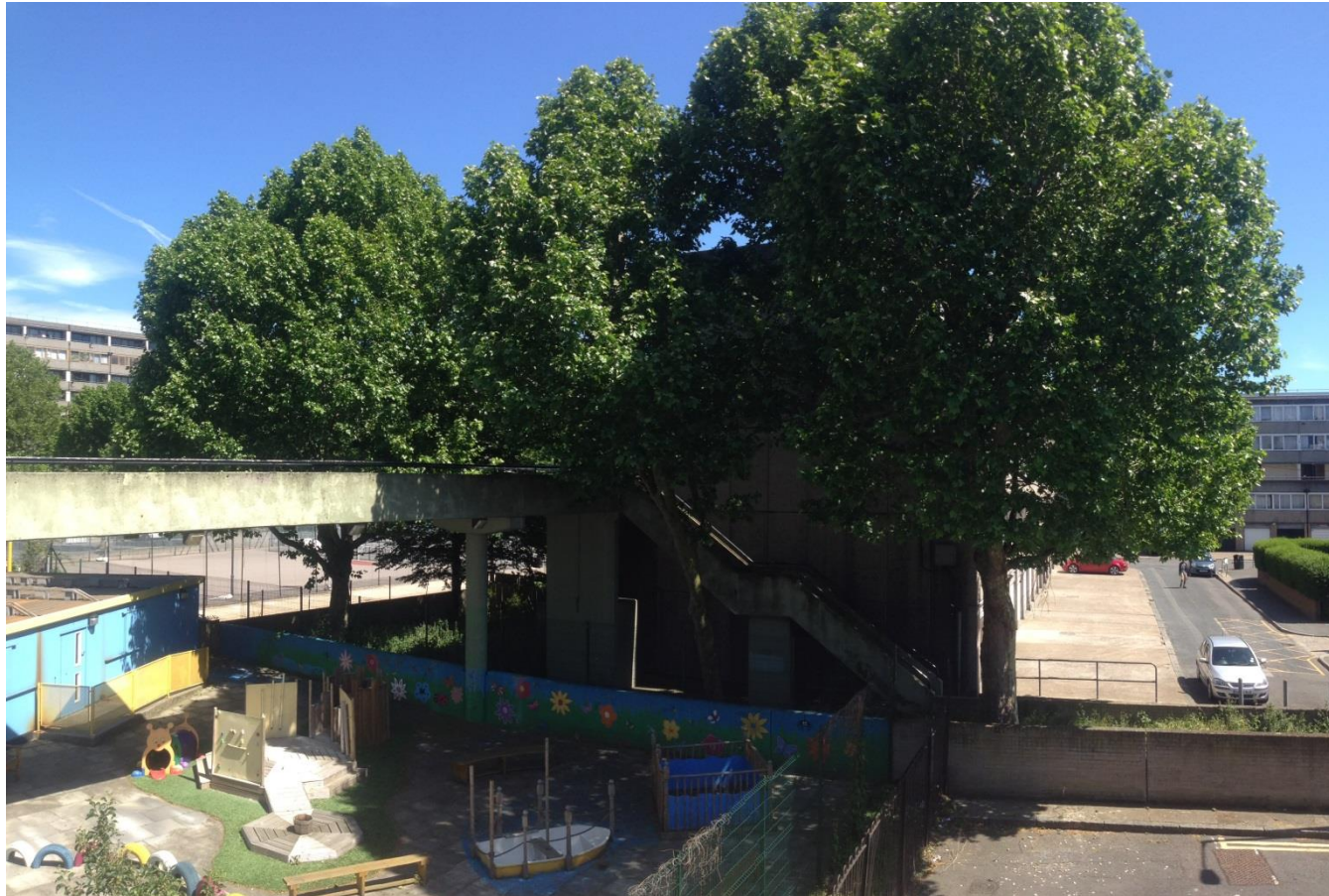
Image 4 – Existing sky walkway to be removed by crane operating from outside RPA areas.
