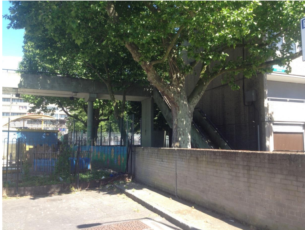
Image 1 – Demolition and replacement surfacing works to be undertaken by hand and under supervision within tree RPA areas
