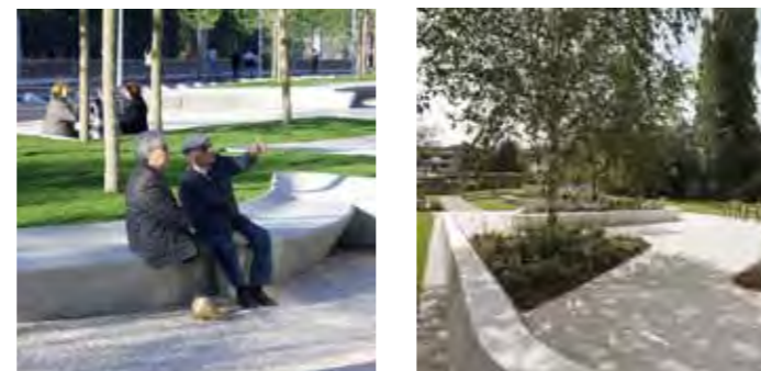
Pre-cast concrete retaining walls to existing trees to be used to create sculptural seating and planting beds
