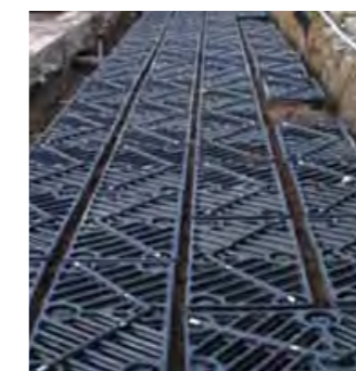
Geocellular soil vault attenuation system used in tree planting
