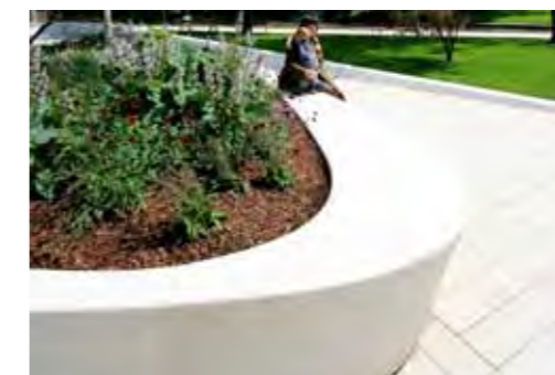
Light acid etch precast concrete with curved profile
