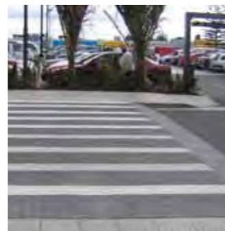
Crossing points to be paved with a consistent material to act as a visual cue to drivers to lower speed.
