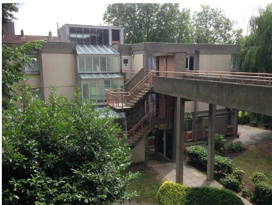
Figure 4: Ellison House and connecting in situ walkway.
