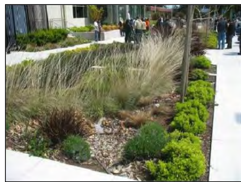
PROPOSED HARD ENGINEERED BIO RETENTION AREA, PROVIDING UPSTREAM SURFACE WATER RETENTION AND WATER QUALITY TREATMENT PRIOR TO DISCHARGE INTO PROPOSED SURFACE WATER SEWER
