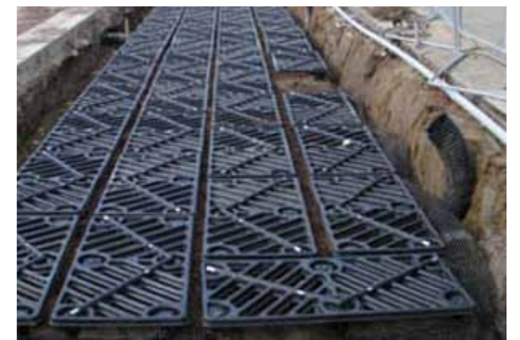
Engineered Tree Pit Attenuation
