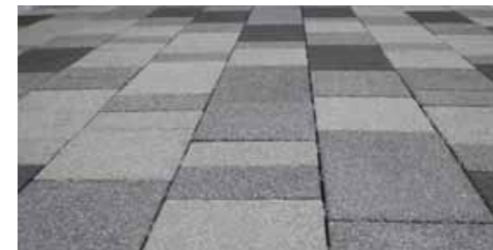
Mixed mid and light grey concrete block pavers
